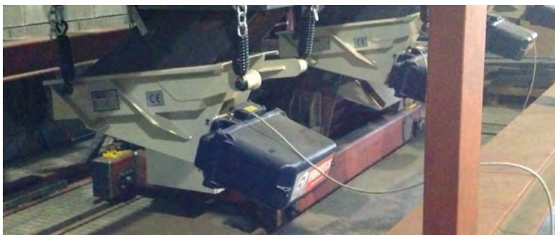
Installation de ferro-alliages
